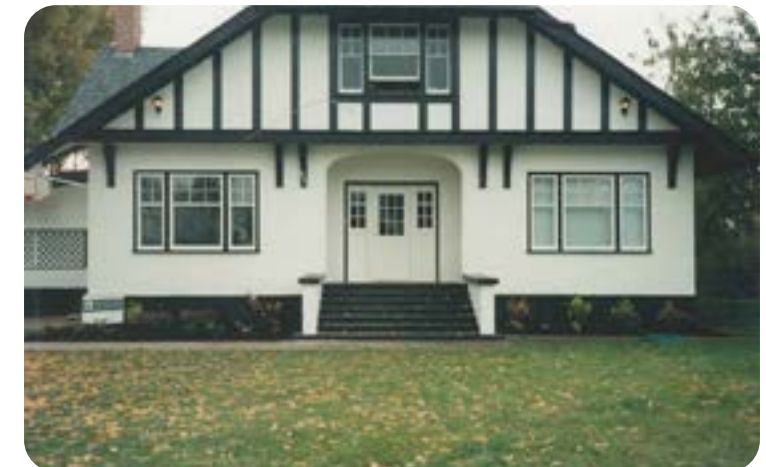
Lawrence Avenue group home closed 2010.
